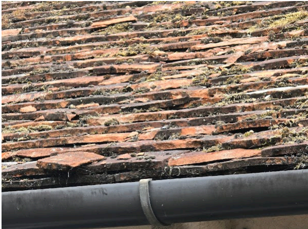
Close up of slipped tiles
