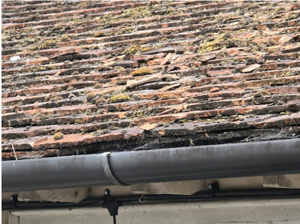
Close up of broken tiles
